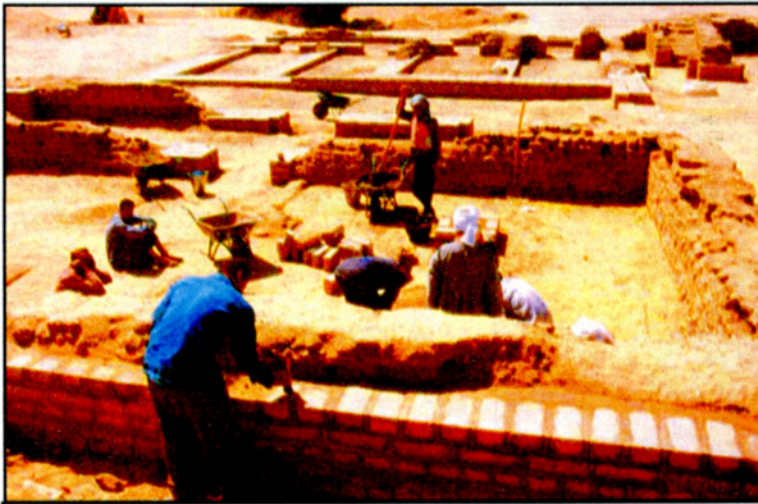
North Palace - Rooms north of the central columned hall during repairs. March/April 2002
